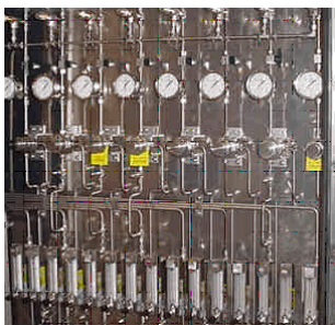
PurgeMaster 10A6100 in liquid sampling panel
